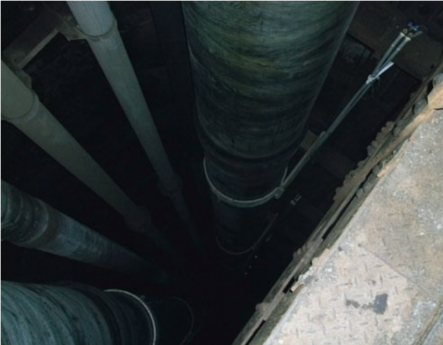
Cladding pipes in place with support brackets fitted
