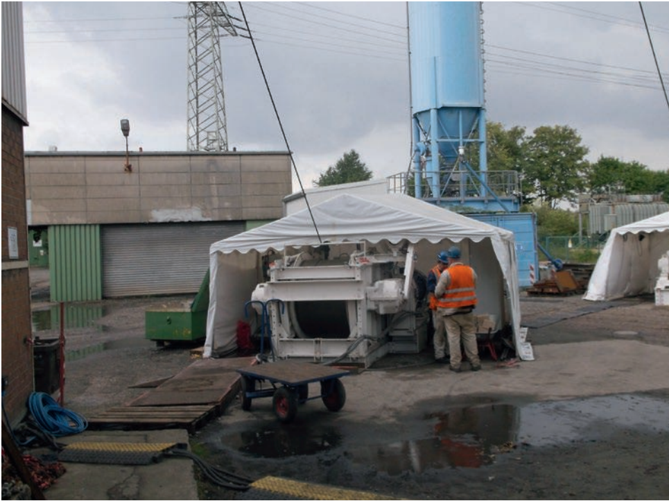
Site preparations – the situation above ground
